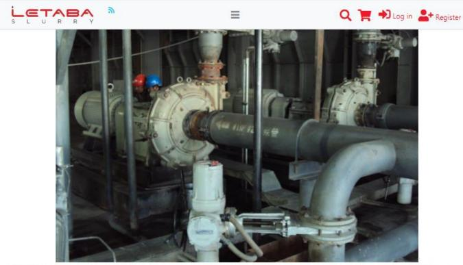
PUMP CONDITION ASSESMENT IS DONE BY A LETABA RELIABILITY ENGINEER/SPECIALIST, THE PUMP IS OPENED AND WEAR ON PARTS IS DETERMINED AND MEASURED WHERE POSSIBLE. THIS IS DONE TO GET AN INDICATION ON THE LIFE LEFT OF COMPONENTS AND TO SCHEDULE REPLACEMENT OF WEAR COMPONENTS.
